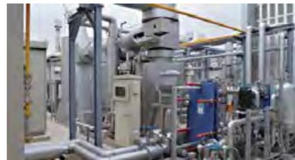
An environment-friendly cogeneration system using natural gas at our Gunma Factory
